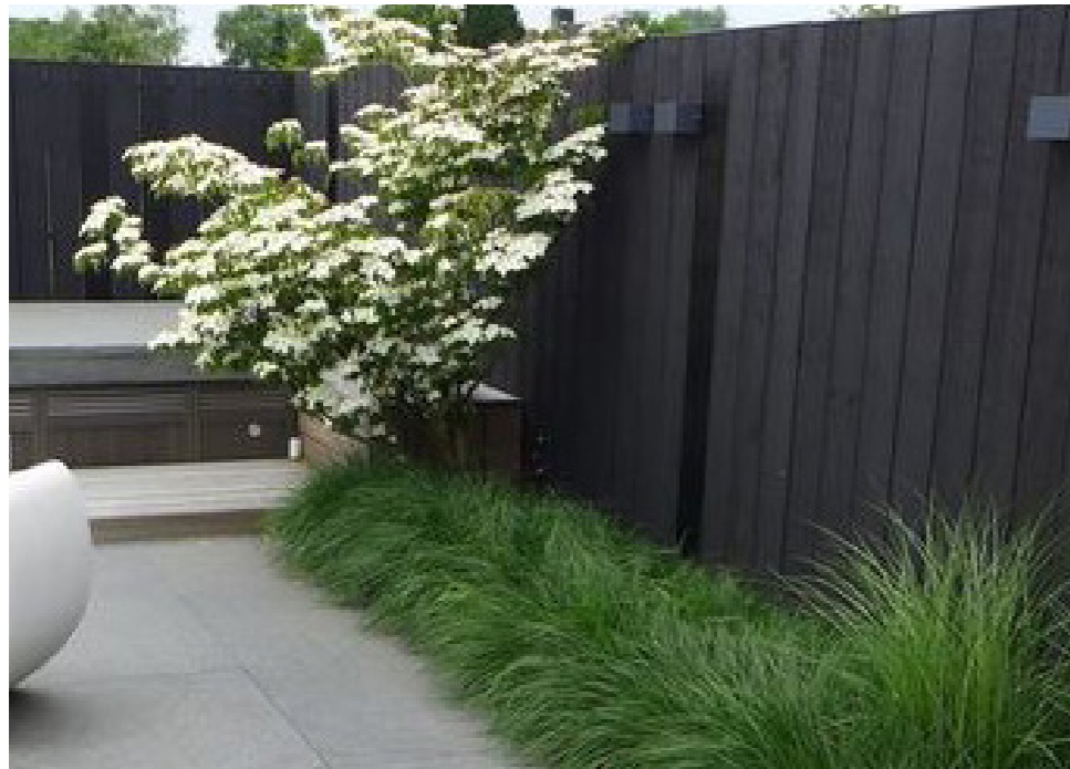
--- Fence type 01 - 1.8m high closed board vertical timber paling fence, stained black/dark grey
